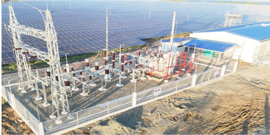
40 MW DC Limbauan Solar Power Project 69 kV switchyard
